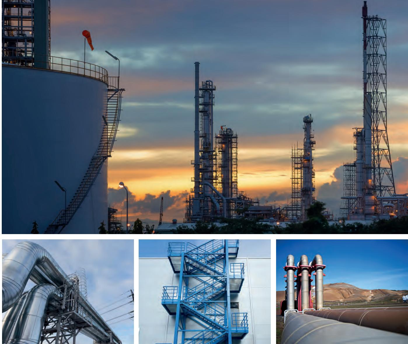
**C5** is subdivided into **C5-I for industrial areas** and **C5-M for marine areas**. Both subcategories correspond to the highest corrosion protection in very aggressive environments. High coat thickness and high-quality two-component coating systems have to be used.
